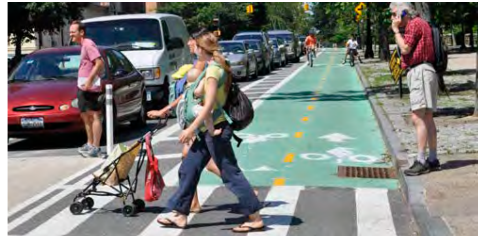
Parking protected "cycle track" Or protected bike lane
