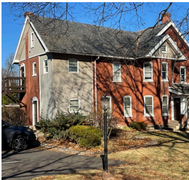
Building addition to the rear of the Sojourner Executive Suites in Harleysville, Lower Salford, Montgomery County.
