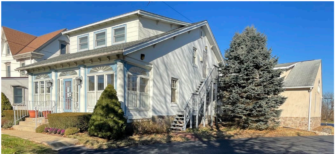
Building addition to the rear of the Pillars of Light and Love property in Trappe Borough, Montgomery County.
