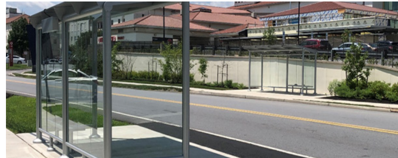
Recently installed bus shelters along Marshall Street serving Chester County Hospital.
