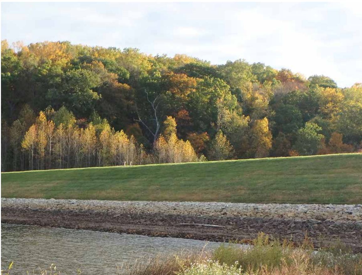
Maintaining and improving flood control infrastructure and minimizing disturbance of floodplains are essential measures for protecting public safety and natural habitats.
