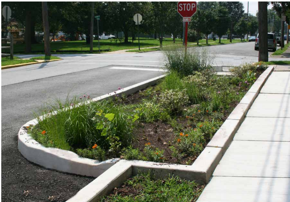
Progressive stormwater management facilities, such as this vegetated curb bump-out in West Chester, can serve as models for reducing stormwater and polluted runoff and enhancing groundwater recharge.
