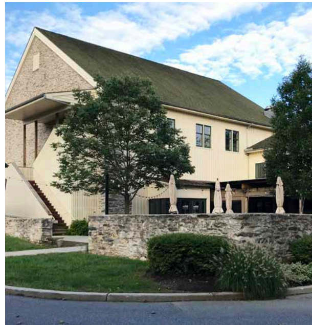
Adaptive reuse of this barn in West Whiteland Township preserved a local landmark and provides a sense of place within new development.
