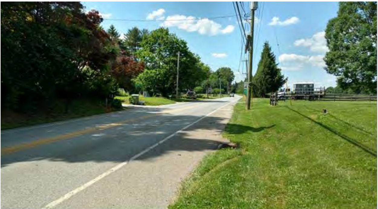
Figure 32. Unionville Road (Route 82), view to the north. This portion of the road is immediately north of the intersection with Street Road (CHG).
