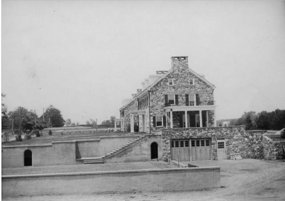
Figure 22. View looking west to the Brewer-Miller House, showing the original wine cellars of the Anvil Tavern, 1918 (P.S. du Pont Longwood photograph collection (Accession 1969.002), Audiovisual Collections and Digital Initiatives Department, Hagley Museum and Library, Wilmington, DE 19807).
