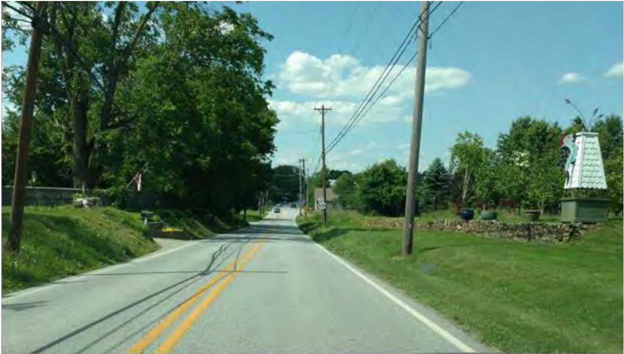
Figure 31. Unionville Road (Route 82) view looking north. This portion of the road is south of the intersection with Street Road (CHG).
