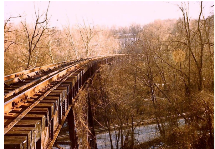
Bridge over PA 29 along Devault Line (Source: TMACC).
